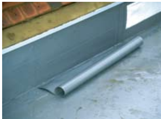
Fig. 3: Edge restraint with alkorPLUS® 81170 metalsheet
