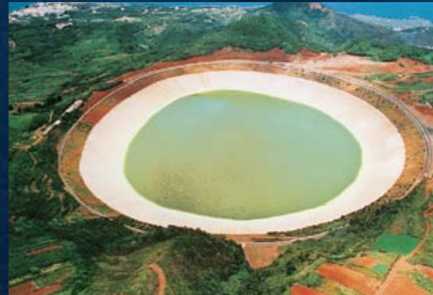
Barlovento reservoir (Canary Islands)
